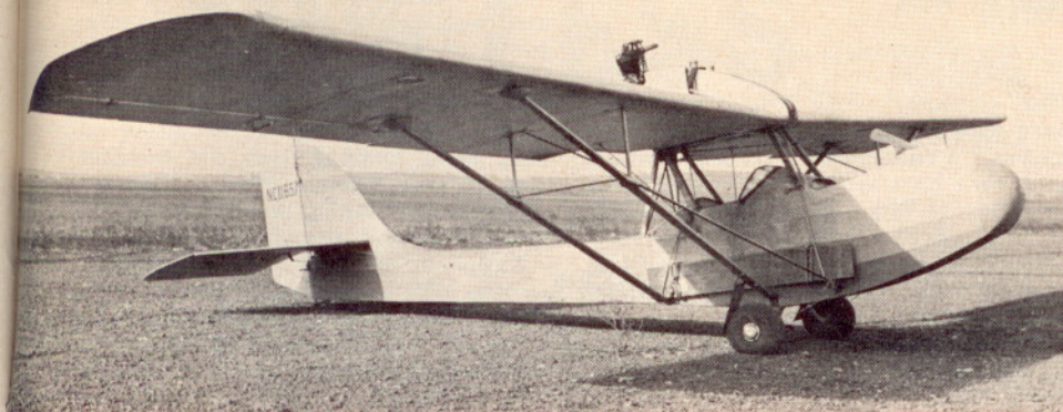
Standard Curtiss-Wright Junior of 1931 used drag strut to replace wire as a required modification. Note external cargo roped to fuselage
